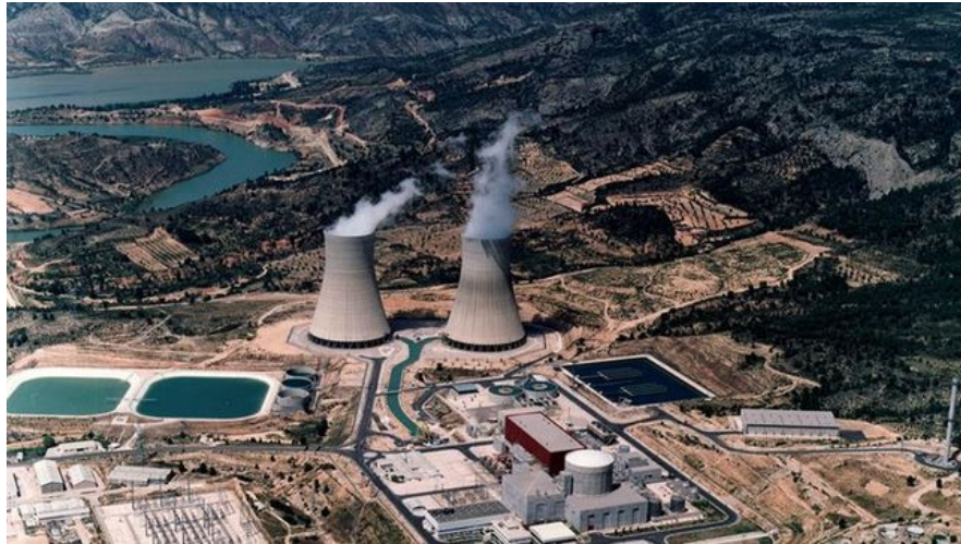
Cofrentes Nuclear Plant (1064 MW) / Cofrentes, Valencia, Spain.
